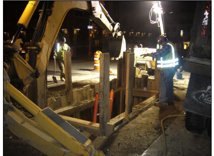
Workers perform nighttime electric relocation work on 2nd Avenue
