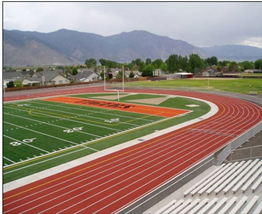
Douglas High School Sports Facility
