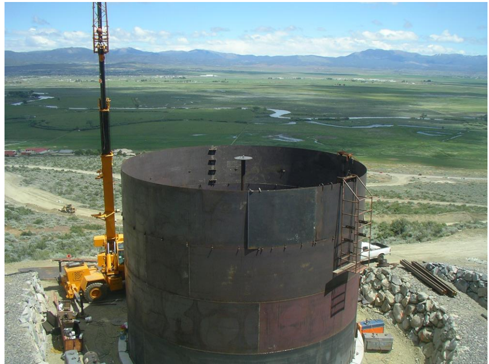
Eagle Ridge Water Storage Tank
