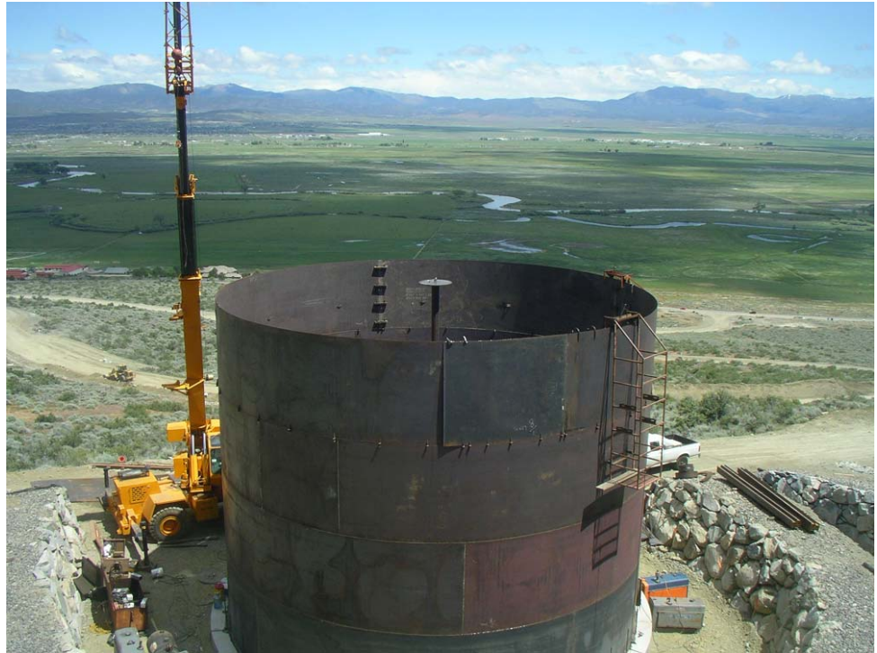
Eagle Ridge Water Storage Tank
