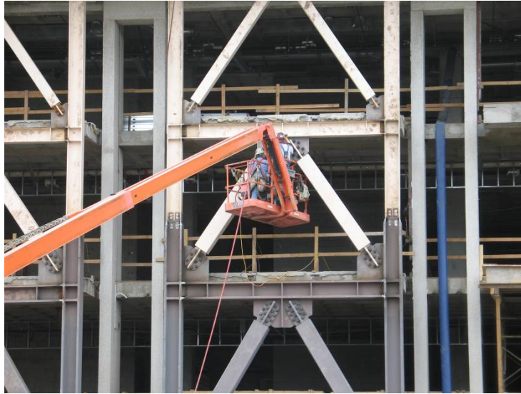
Figure 5: Unbonded steel braces are used as part of the seismic rehabilitation of the Library on the University of Utah campus. (Courtesy of Kelly Peterson, University of Utah)
