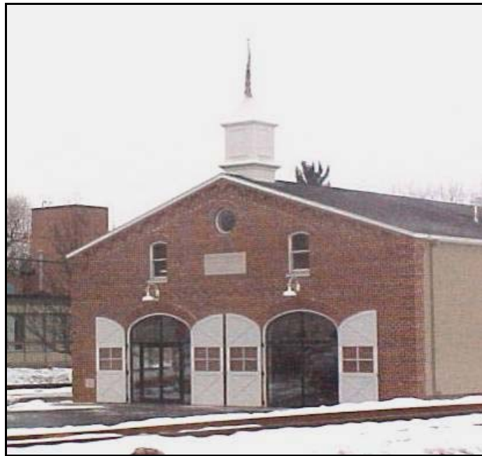
Figure 8: Lewisburg, PA Fire Station. (Courtesy Shubha Shrivastava)
