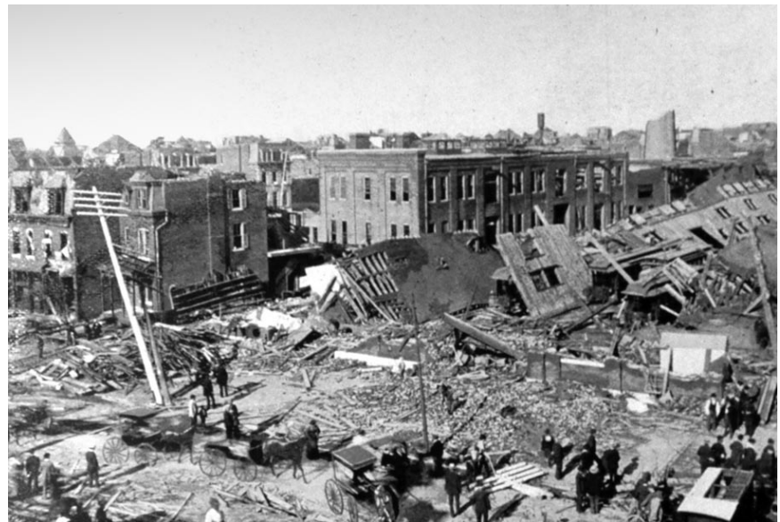
Jefferson and Allen Avenues, St. Louis, Missouri, after the tornado, May 27, 1896.
