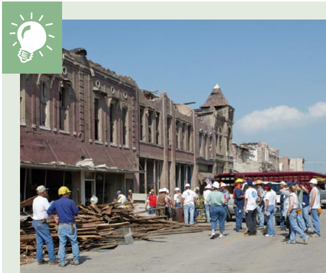
In the wake of a series of tornadoes, many of Pierce City, Missouri's commercial historic buildings were heavily damaged.
