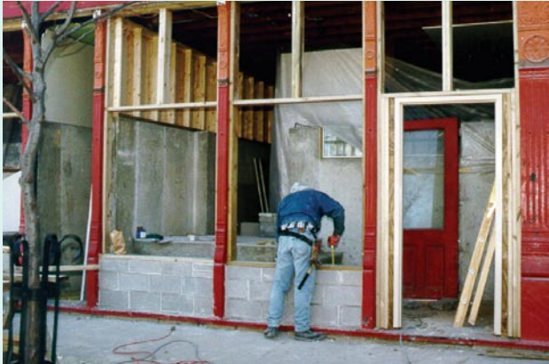
Top: Restored and retrofitted building. Middle: To provide additional protection against floodwater, removable watertight floodgates were incorporated into the buildings. Bottom: Floodproofing in action in Darlington, Wisconsin.
