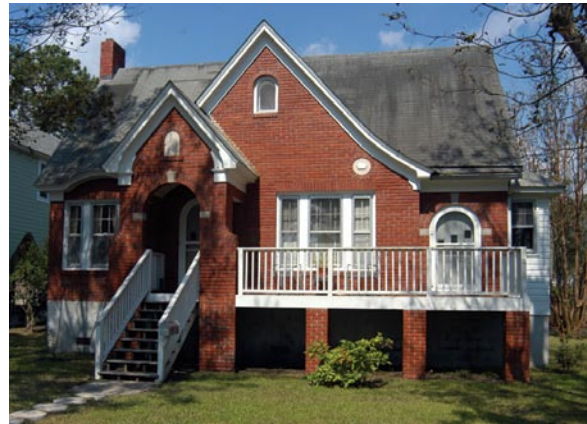
Frame building elevated on concrete block foundation faced with brick veneer. Belhaven, North Carolina.
