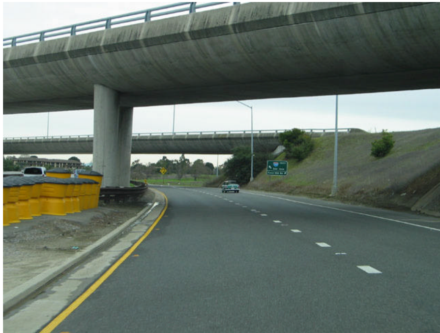
Figure 4-9: Typical overpass that causes total satellite outage and results in high GPS errors
