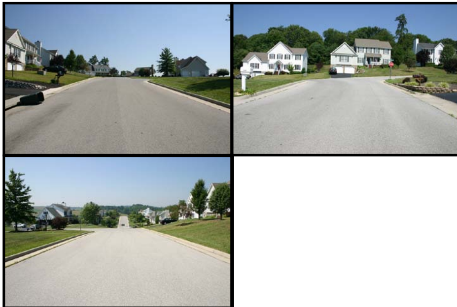
Figure 35 Ground images of Independence & Sapphire intersection.
