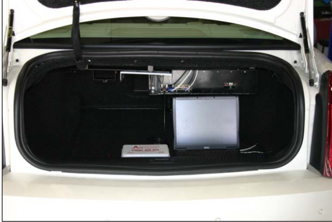
Figure 8 Data Acquisition System, installed in the vehicle trunk, underneath the rear shelf.
