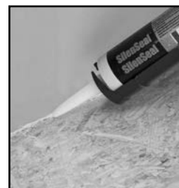
Fill any gap between the wall and subfloor or wall and ceiling with sealant.
