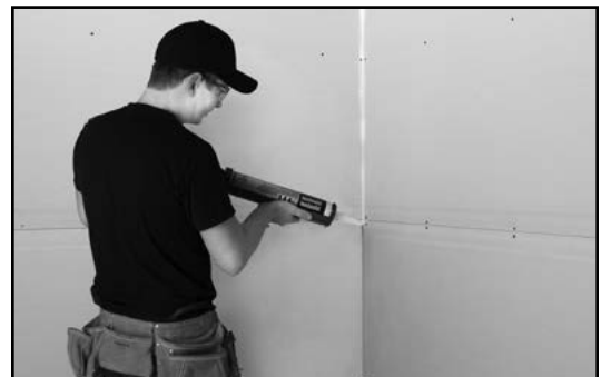
Seal any gap in the rooms corners.
