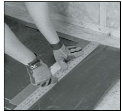
Cut Barrier to the appropriate length.
