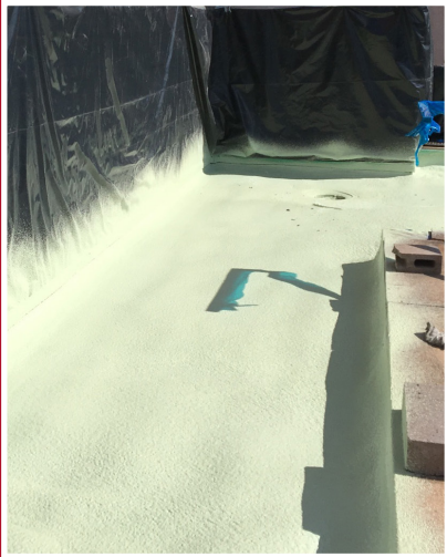
GacoRoofFoam 2733 Closed Cell Spray Polyurethane Roofing Foam.
