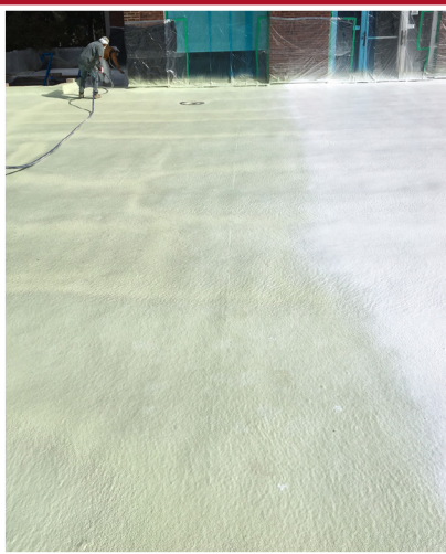
GacoRoofFoam 2733 Closed Cell Spray Polyurethane Roofing Foam being coated with GacoFlex S20 Silicone Roof Coating.
