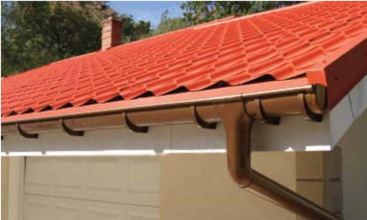
*Galata Chemicals Mark® T650 and Mark® T652, new octyl tin heat stabilizers, are designed to replace butyl tin heat stabilizers used in outdoor PVC applications such as corrugated sheet, coextruded sheet and rain water guttering.*
