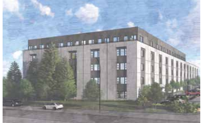
The Notable (730 Simms) project in Lakewood, CO is an example of a 218-unit affordable housing development partially financed with a private placement of tax-exempt bonds.
