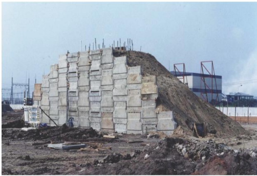
THE FINISHED 6M HIGH REINFORCED EMBANKMENT
