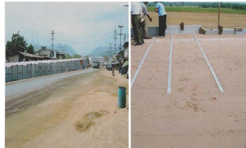
MSE WITH STEEL STRIP REINFORCEMENT
