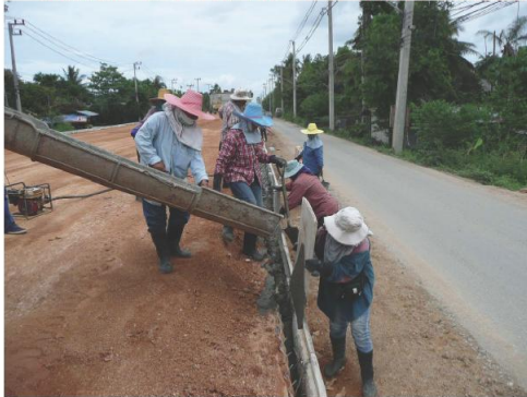
MORTAR FILLING OF FACING AT RIGHT APPROACH
