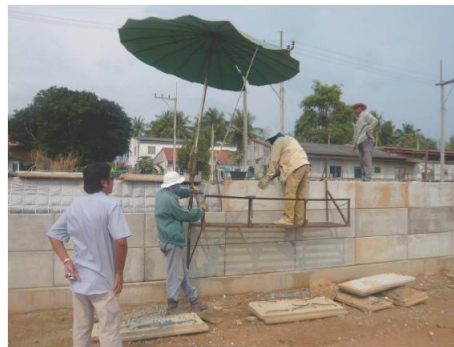
CONCRETE FACING INSTALLATION STA.8+000 (FINISHING APPROACH BRIDGE)
