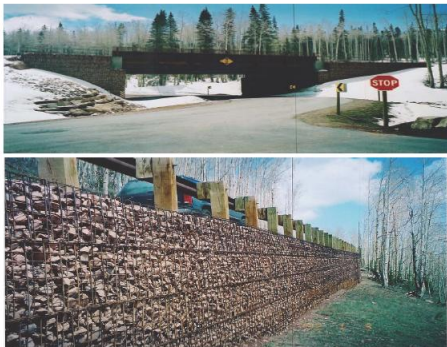
HILFIKER MSE WALL WITH STEEL GRIDS REINFORCEMENT IN PARK CITY, UTAH
