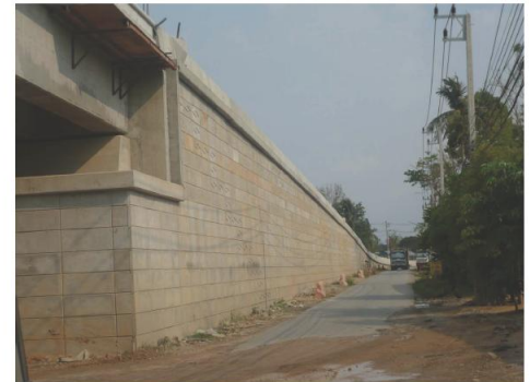
SIDE VIEW OF MSE WALL STA. 4+000 (FINISHING APPROACH BRIDGE)
