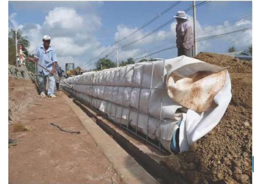
COMPLETION OF 1 ST GRID LAYER
