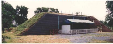
Steel-Grid MSE Embankment on Unimproved Soft Clay Foundation
