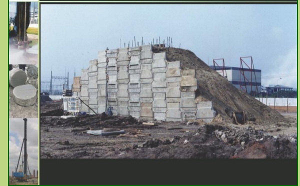
The Finished 6m High Reinforced Embankment
