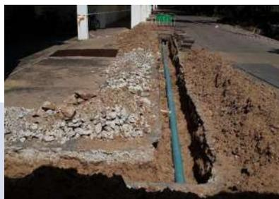
**REPLACEMENT OF WATER PIPELINE FROM ADMIN BUILDING TO WATER TOWER**
