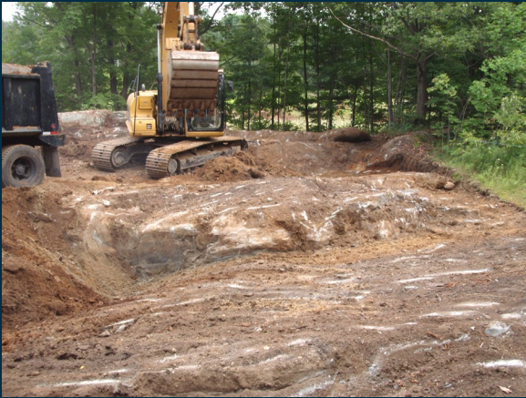
Isolating piles of impacted soil for treatment with biomix
