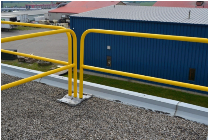
Figure 7: Two Edge Rails with Tieback Rail
