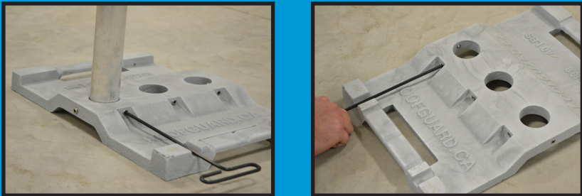
Figure 8 & 9: Installation of Baseplates
