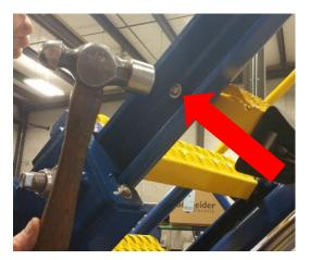
6. Tighten up hardware with a 9/16 ratchet and 3/16 Allen Key
