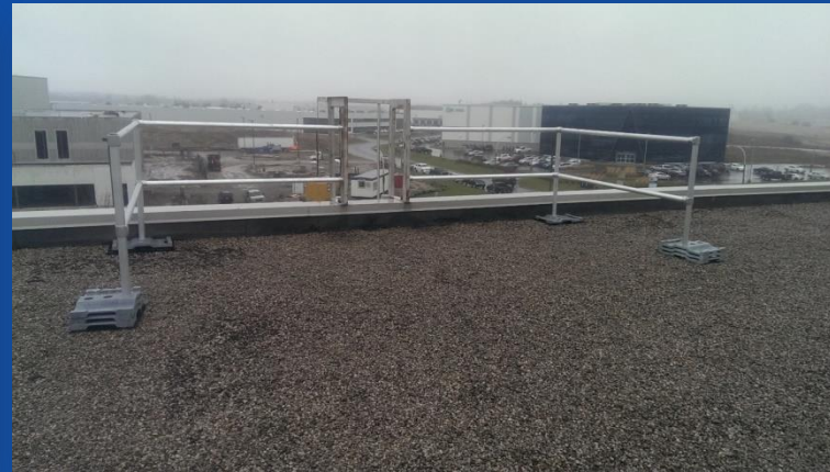
RoofGuard system attached directly to fixed access ladder to allow for safe access to ladder – provides a safe work zone for entry and exit from ladder to allow workers to get out onto the roof surface safely without getting into the 6 ft zone near the roof edge.
