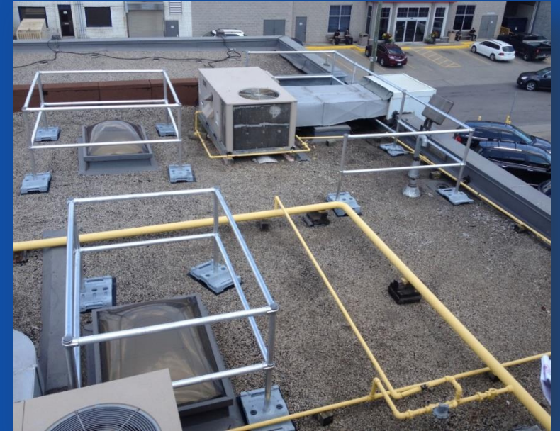
Typical skylight system
