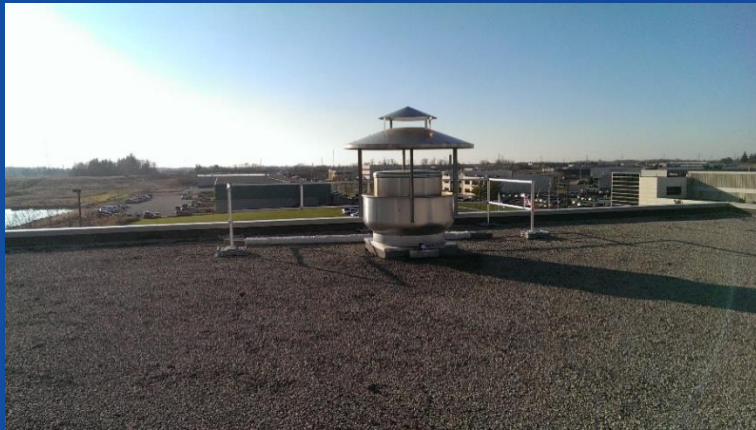
18 ft RoofGuard Kit protecting single mechanical unit
