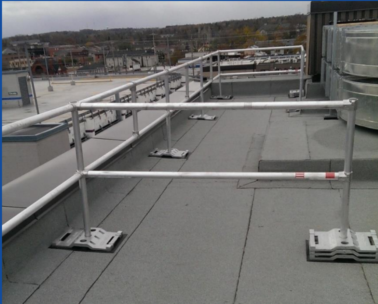
Typical Setup showing 6 ft returns every 27 ft, corner setup with return facing inwards, rubber pads to protect the membrane
