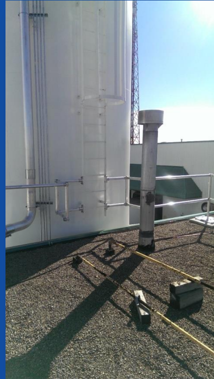
RoofGuard system attached directly to a fixed access ladder to provide complete protection while accessing the ladder
