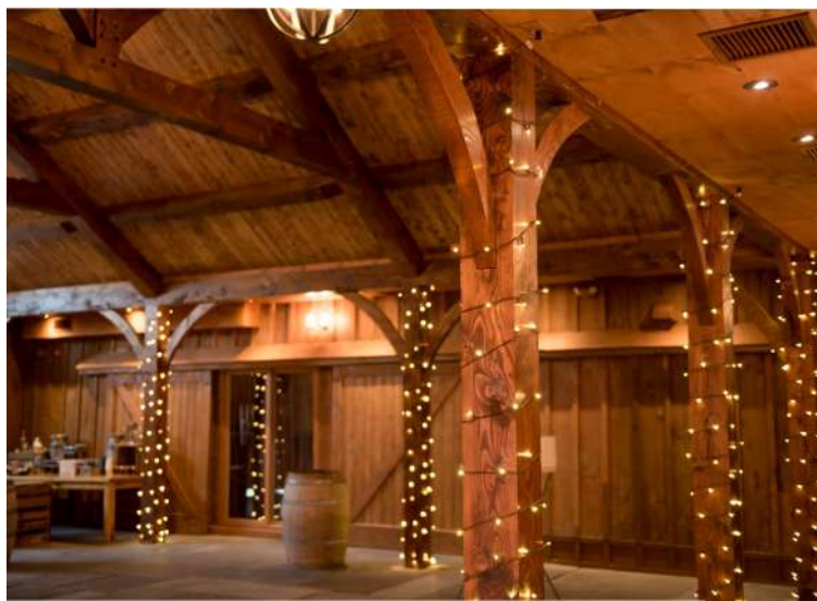
Pin Lights on Columns
