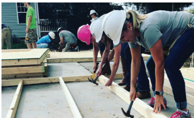
Habitat for Humanity home build
