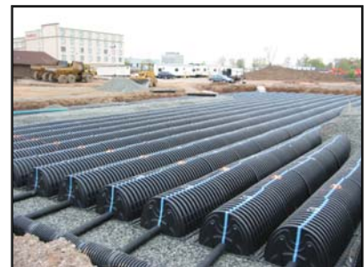
Option #3 - External conventional pipe and fitting manifold
