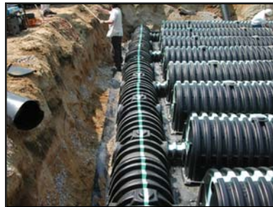
Option #2 - External manifold using CULTEC HVLV® 180 Header System
