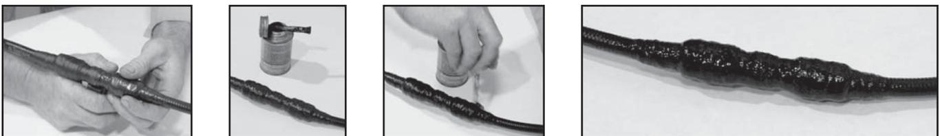
This material works very quickly to fuse the last layer together and to the cable jacket. After the Scotch-Kote has dried, encapsulate the finished connection with the mastic material.
